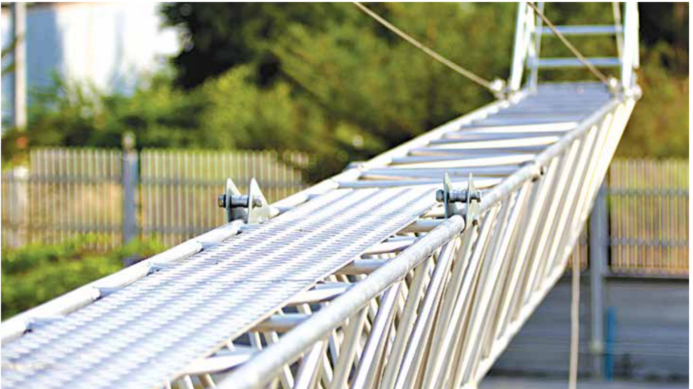
anti-slip aluminium plate on stepping area (PLA-00-0004)
