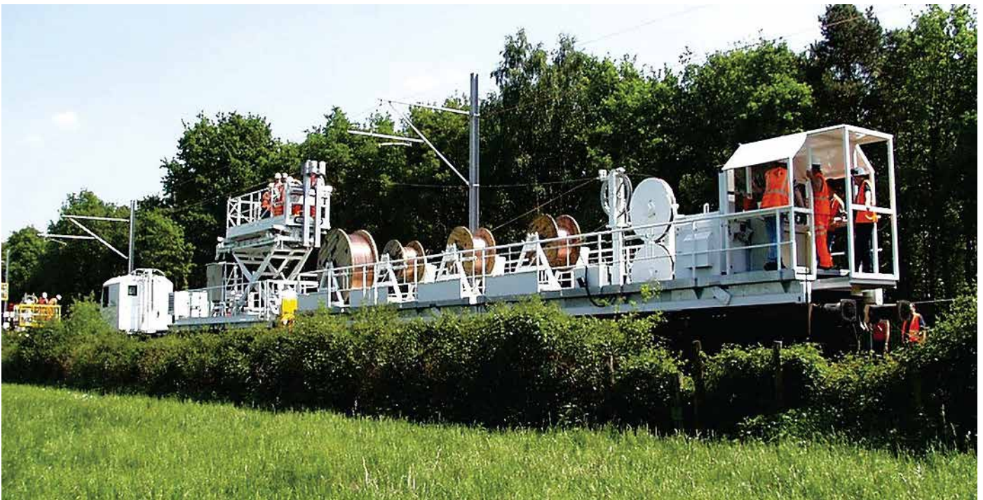
Catenary Installation Unit mounted on self-propelled wagon
