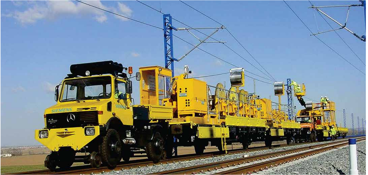
catenary installation unit pulled by rail-road truck
